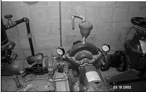
Fire Pump Housing and Gauges
